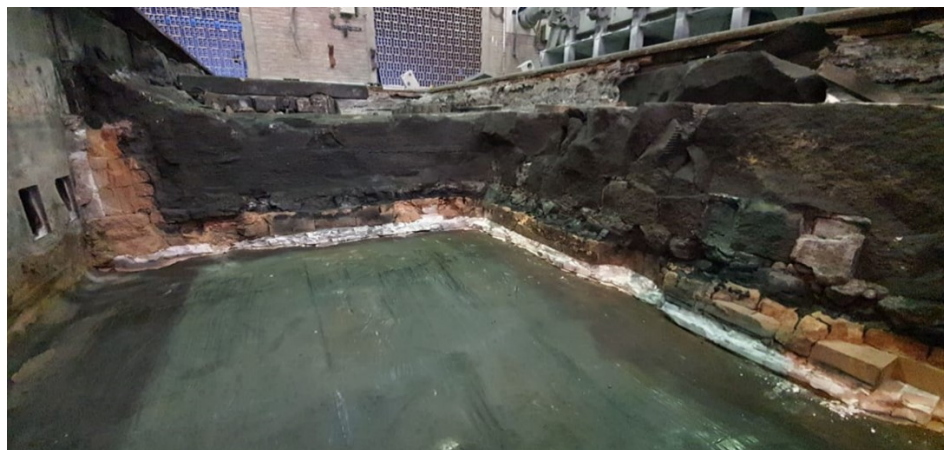
Figure 5. Controlled demolition of the first prototype.
